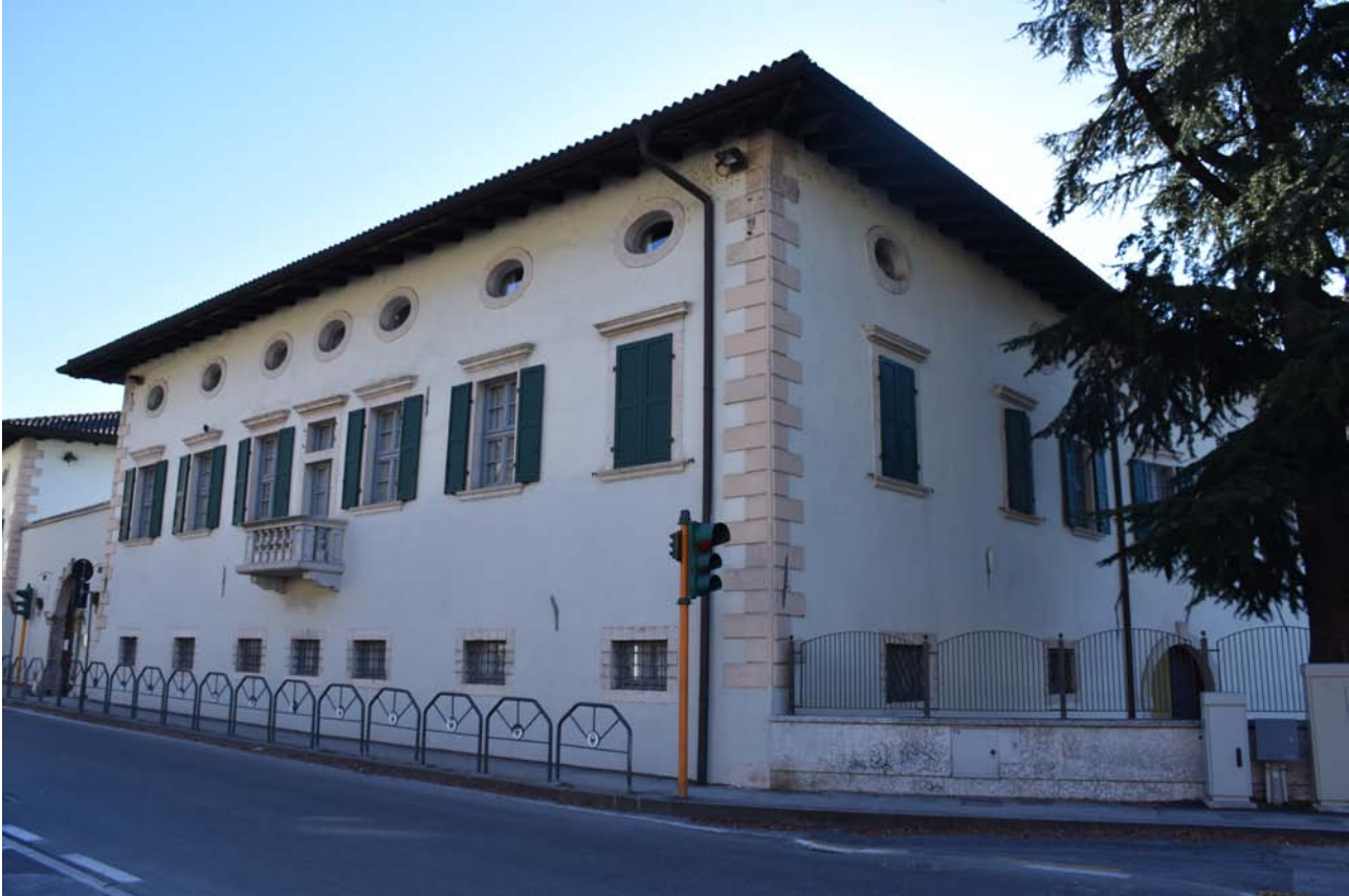
Gardolo – palazzo Crivelli (p.ed. 89 C.C. Gardolo)
